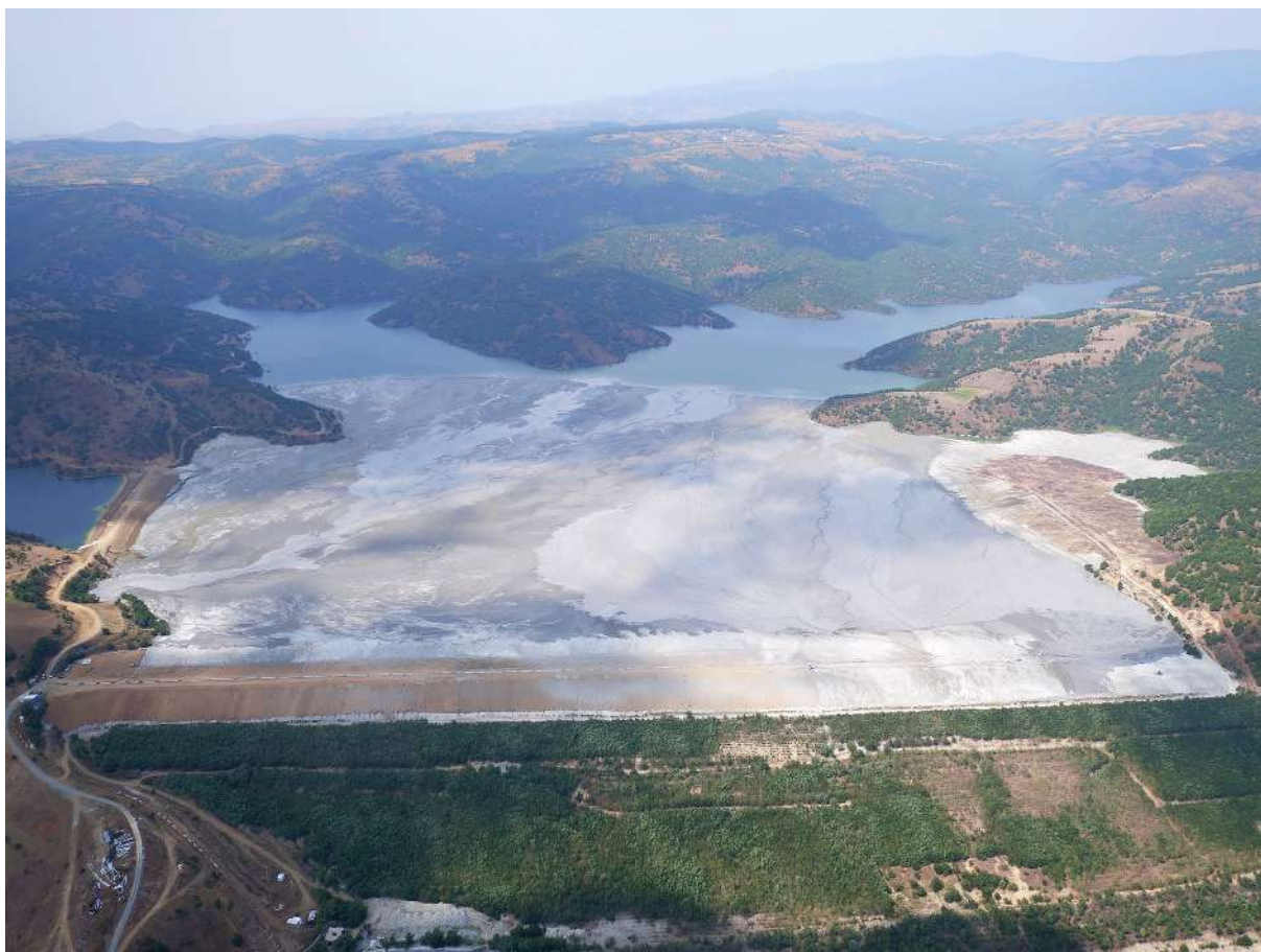
Figure 1: Tailings dam "Topolnica" (Srbinoski et al., 2016–2021).
