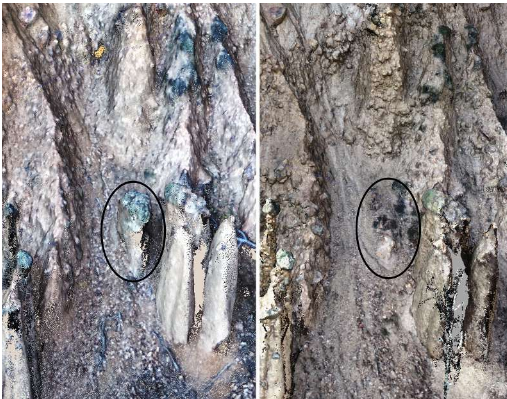
Figure 5: Identification of sinking rock that was on the top of earth pillar between 3D model generated from 2018 mission (left) and model generated from 2024 mission (right)
